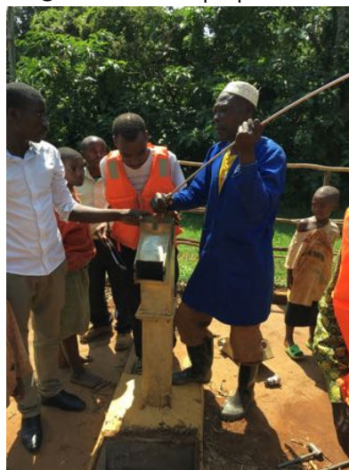
Photo right: Hand-pump mechanic identifies the issue with a non-functional borehole in Rusizi district
